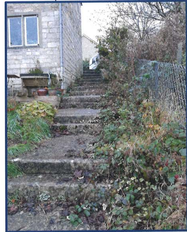
Middle of path looking towards Point A alongside Weavers Row.
