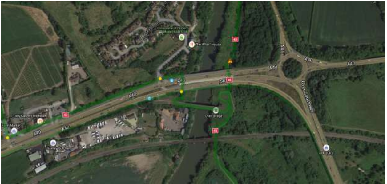
Figure 1.2: A40 Over Roundabout Study Area
